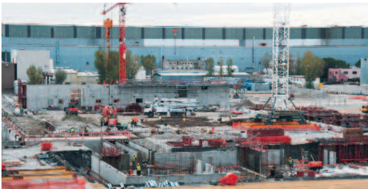
Georges Besse II plant construction site
