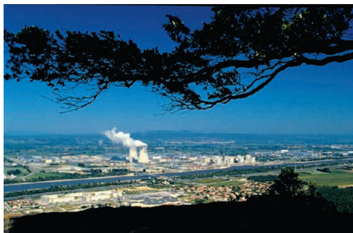
Tricastin site – general view
