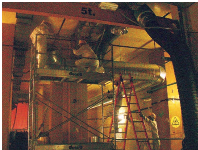
Brennilis – renovation of the ventilation system
