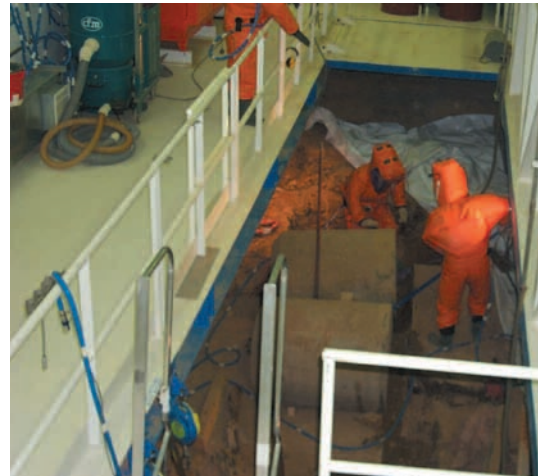
Trench emptying worksite, BNI 56
