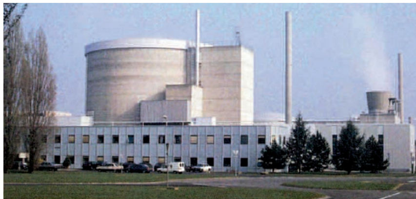
Overview of the ORPHÉE reactor installations
