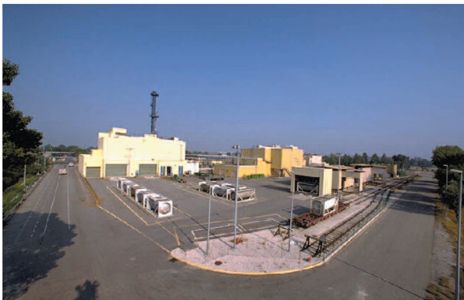
TU5 – general view
