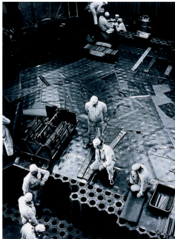
Graphite assembly in graphite gas reactor
