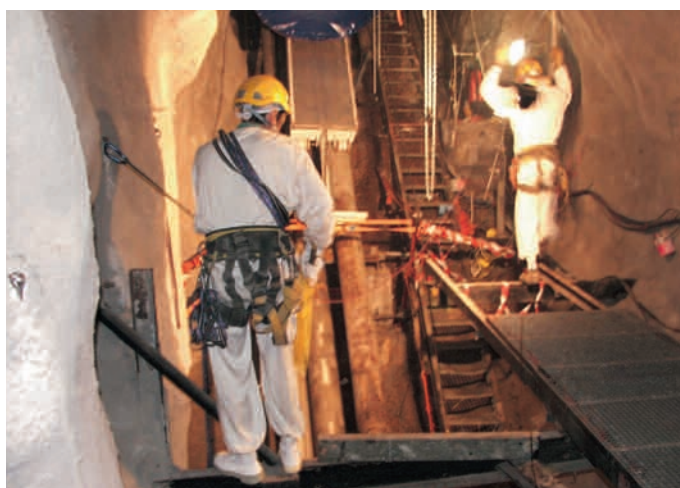
Chooz A – dismantling of ventilation flue
