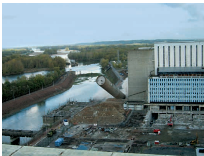
Chinon – blasting of the CHA 3 water tower
